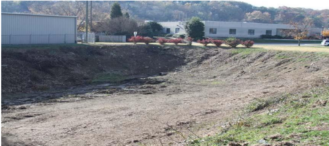
Discharge Control Pond at Operations Center
