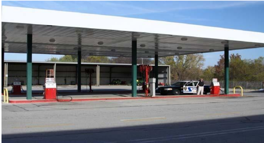
Fueling Center at the Operations Center
