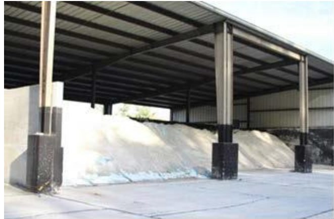
Road Treatment Material Storage at Operations Center
