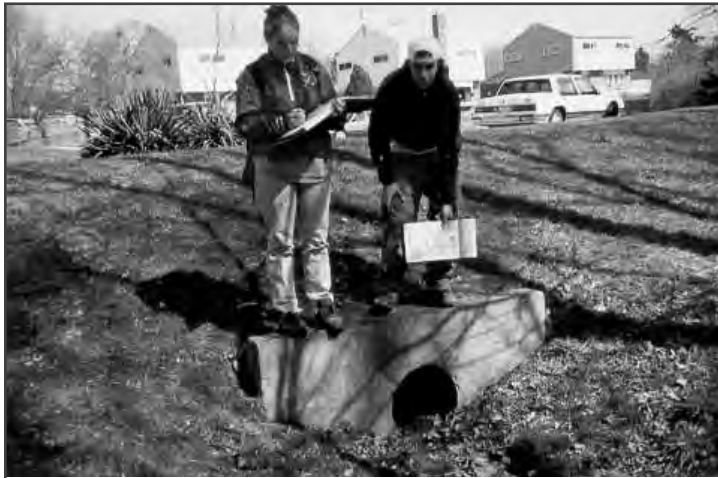
Figure 4.6.4-3. Minor pipe outfall site.
