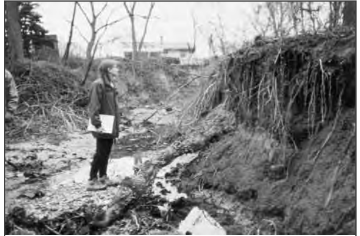
Figure 4.6.2-1. Photograph of a stream erosion site.
