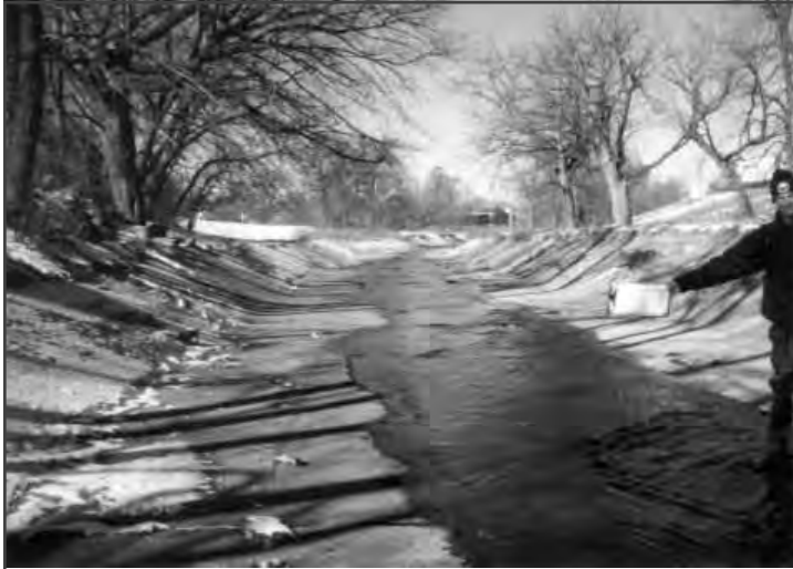
Figure 4.6.1-2. Severe Channel Alteration
