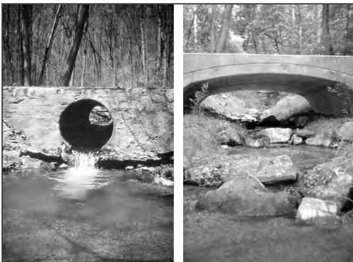
Figure 4.6.5-4. Perched culvert before and after restoration project.
